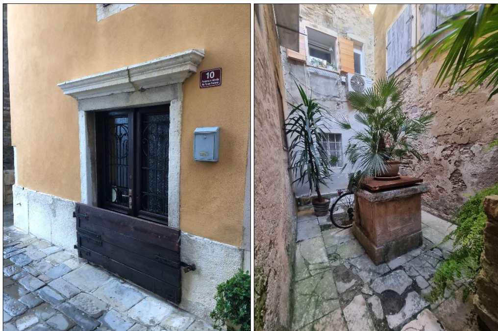
Fig. 1: Left: Example of an anti-flood barrier that has been traditionally used in old-town Piran. / Right: Top part of a stone water well in old-town Piran. The floor on which the water well is positioned, is used as patio, but is basically the ceiling of a cubic water cistern.
