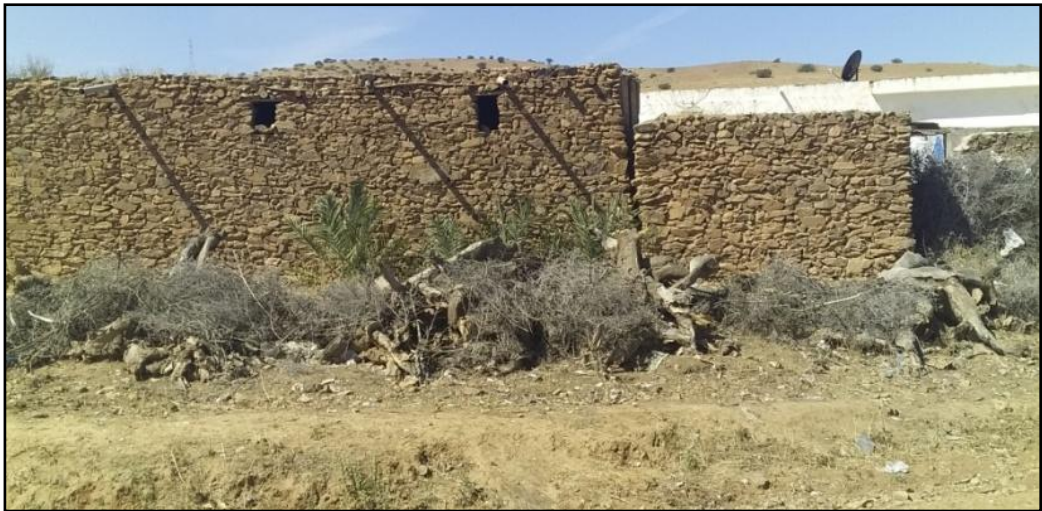
Figure 14: The Schist Housing is built by Locally Extraction Stones in Ouled Jarrar part.
