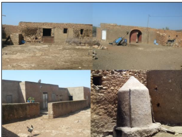
Figure 13: The Traditional Housing is Built by the Limestone Stones in Doukkala Area. Source: Field work, 2024.
