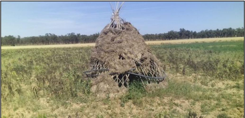
Figure 8: The Noala is Covered with the Reed and the Hay in Doukkala East.
